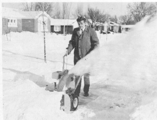
ARIENS SNO-THRO Self propelled, 2 stage, heavy duty 3½ h.p. or 6 h.p. rotary snow thrower. 180° swiveling SNO-CHUTE with hand crank directional control.
